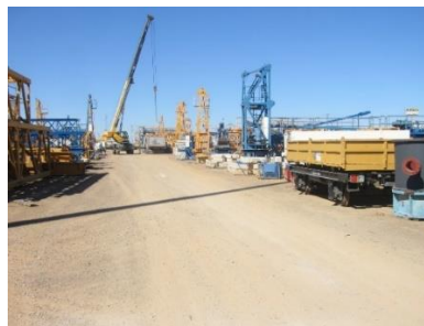
PICTURE IRSIPAA 5 ACCIONA CONSTRUCTION SA EXTERIOR AREA
